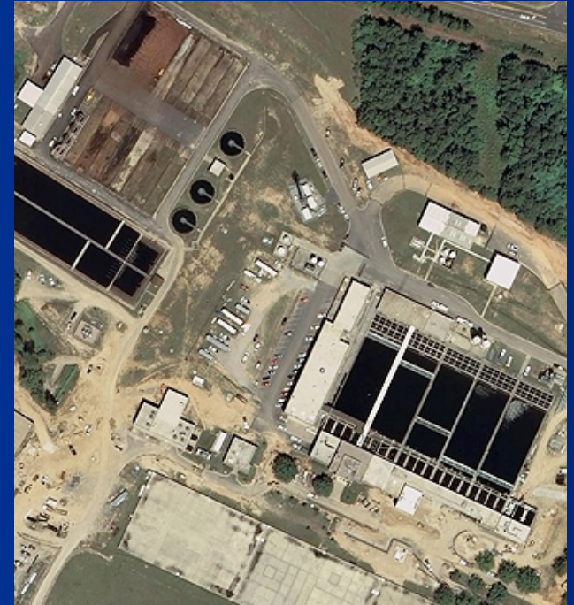
E.M. Johnson water treatment plant, Raleigh. Photo: Hazen & Sawyer
